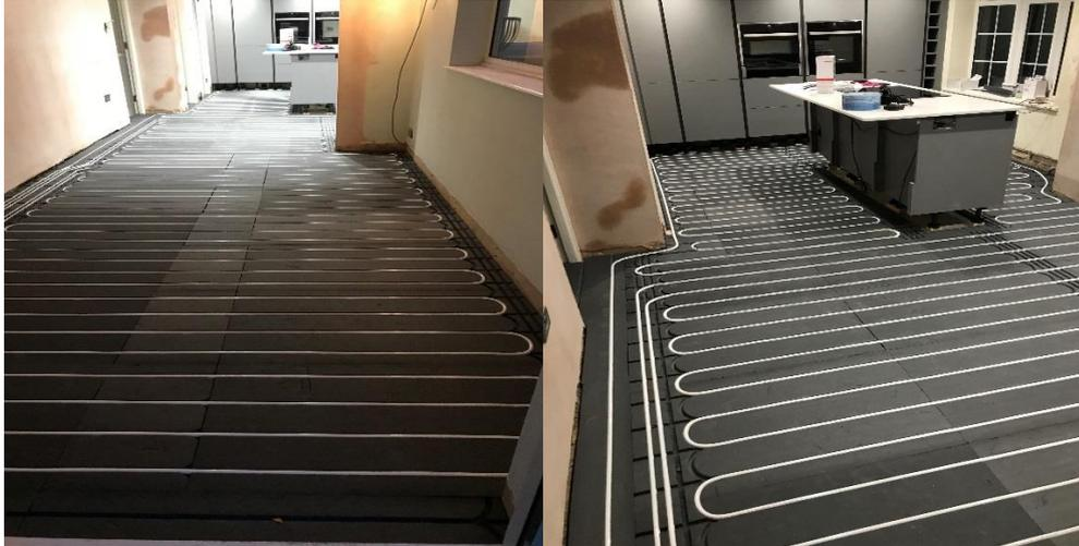
10. If there's a point where the pipe isn't sitting flush in the groove, use a pipe clip and cut it into the board. The board can be cut with a trimming knife or hot wire and material removed to create pipe grooves.
