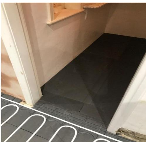
12. Use grip rails where pipe congests near the manifold and we recommend the void is filled with levelling compound before floor coverings are fitted.
