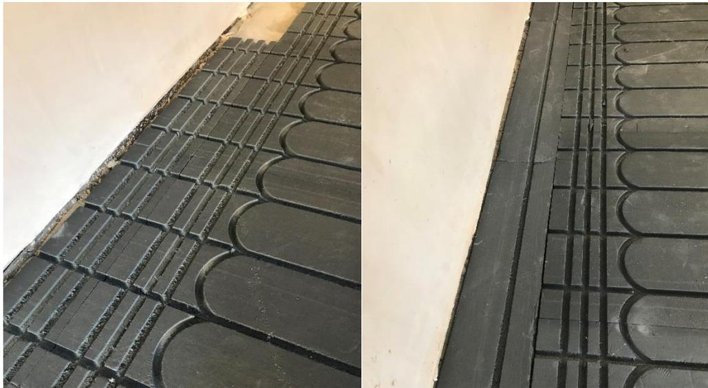
4. Once you are satisfied that the boards are in the correct position for the pipe, number the boards on the upper face to identify the position of each board. This will help when fitting the boards in place after priming etc.
