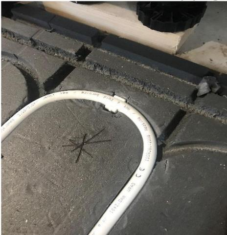
11. 'Blank' boards can be used for areas where UFH is not used.
